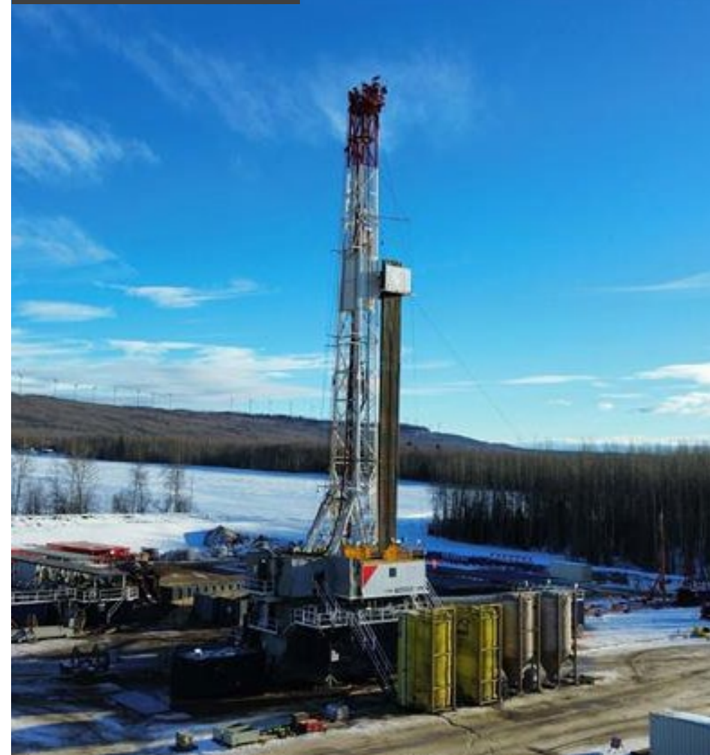
Tupper Montney – Drilling Rig
